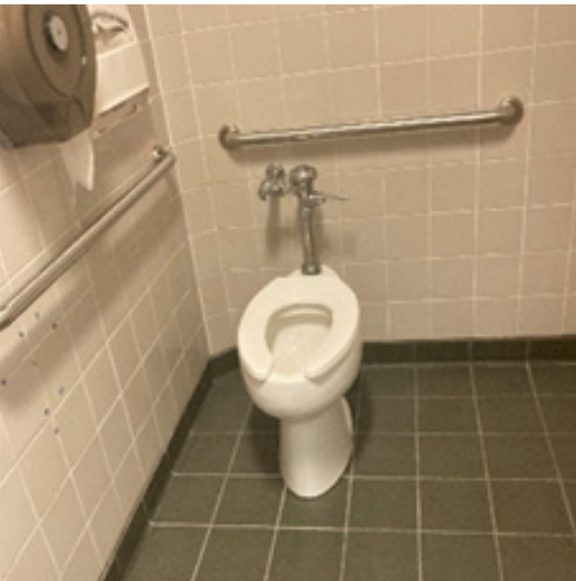
Fig P-24 - Water Closet at ADA Restroom
