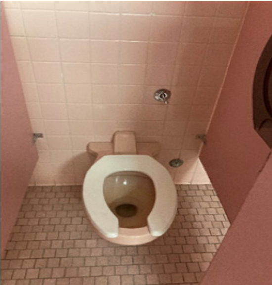
Fig P-14 - Water Closet at Women's Restroom
