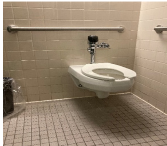
Fig p-10 - Water Closet at ADA Restroom
