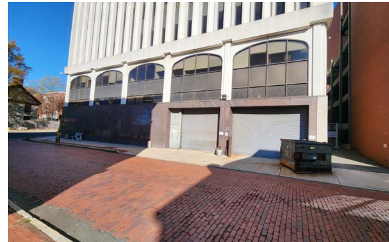
Photograph 4: South side of the building. Brick streets in this area need repair. Street trees area missing.
