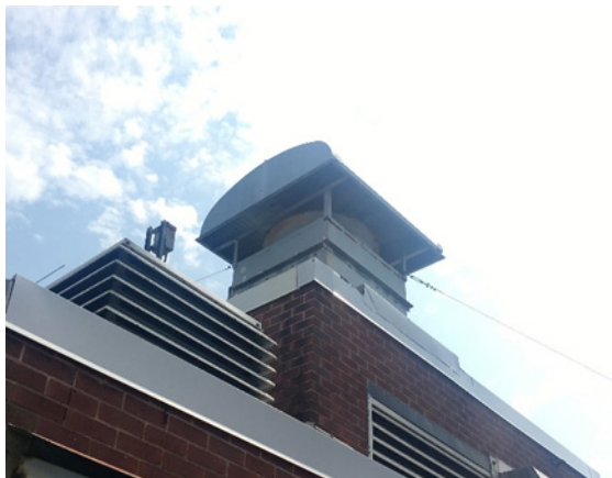
Fig H-10 - Typical Stairway Pressurization Fans
