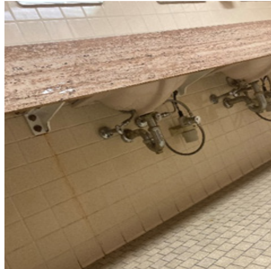
Fig P-18 - Lavatory Drain Assembly
