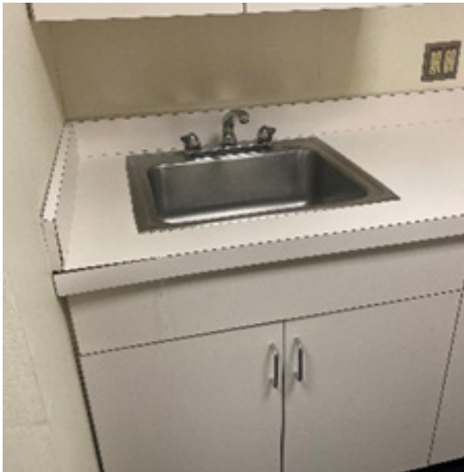
Fig p-25 - Kitchen Sink
