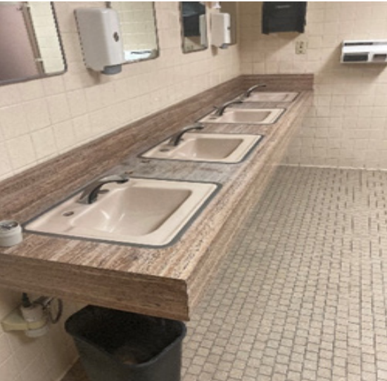
Fig P-17 - Lavatories at Men's Restroom
