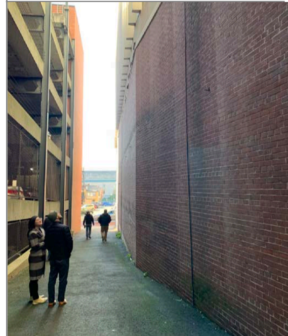
Photo 1: Alley at the east side of the building
