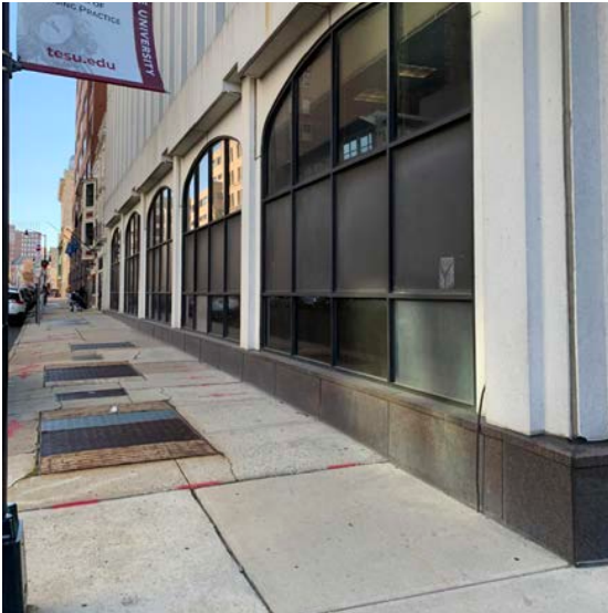
Photograph 2: North side, along West State Street. Concrete sidewalks with grates for below grade transformers.
