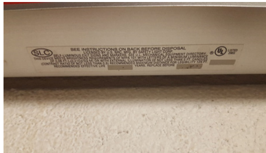
Fig E-10 - Illegible Labels on Exit Sign for Life Expectancy and Expiration Date
