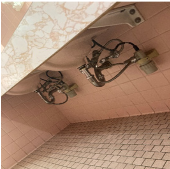
Fig P-13 - Lavatory Drain Assembly
