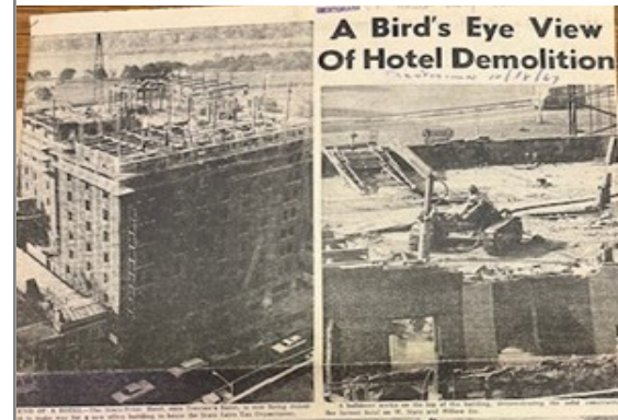
Trenton Times newspaper story from 1967 regarding the demolition of the Stacy-Trent Hotel
